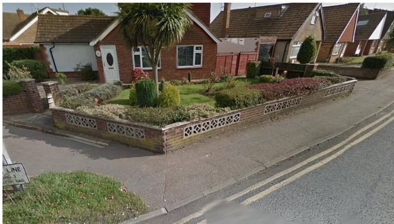
Image 6: View looking at the existing kerblines with little to no upstand on Cloes Lane
